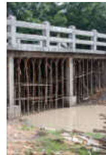
The bridge is almost finished, just in time for the rain.
