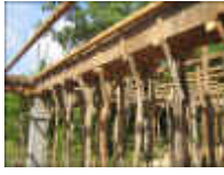
Preparing the span.
