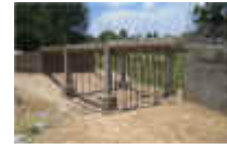
Looking more like a bridge.
