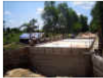
Ready for concrete.
