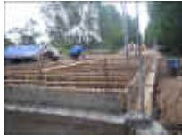
Timber for the formwork was one of the major expenses.
