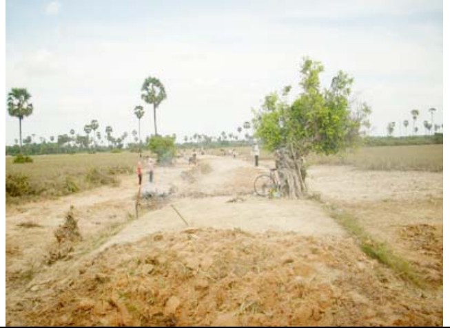
The partly completed road.
