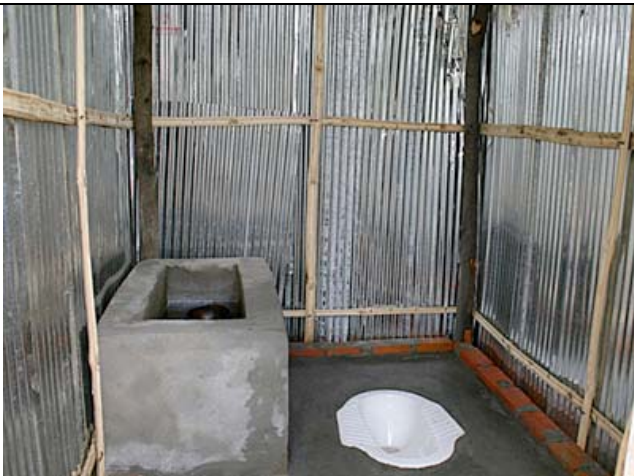
Inside one of the toilets built as part of our sanitation project.
