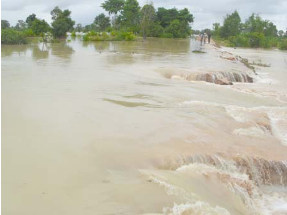
A road being destroyed by the fast moving water.
